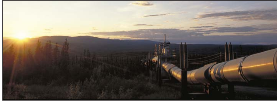
The trans-Alaska oil pipeline
