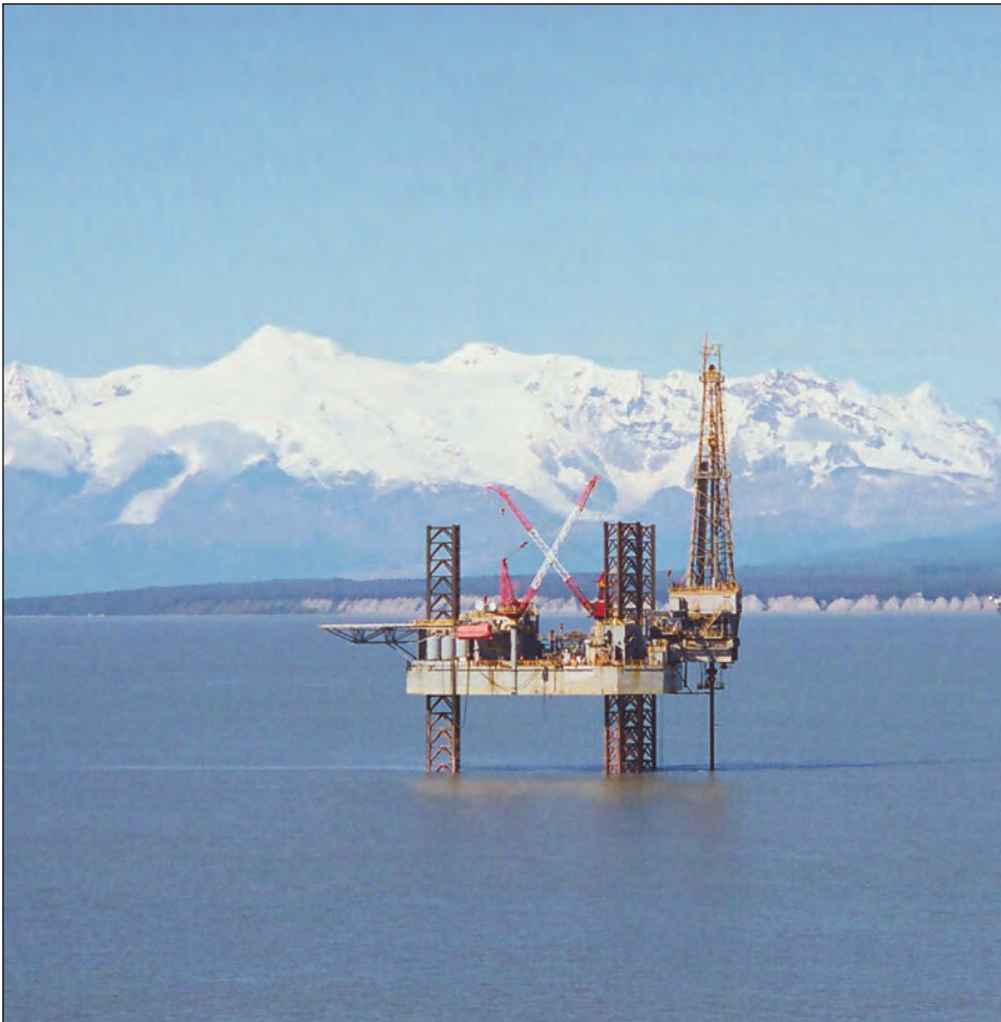
The Spartan 151 is an independent leg cantilever jack-up rig
