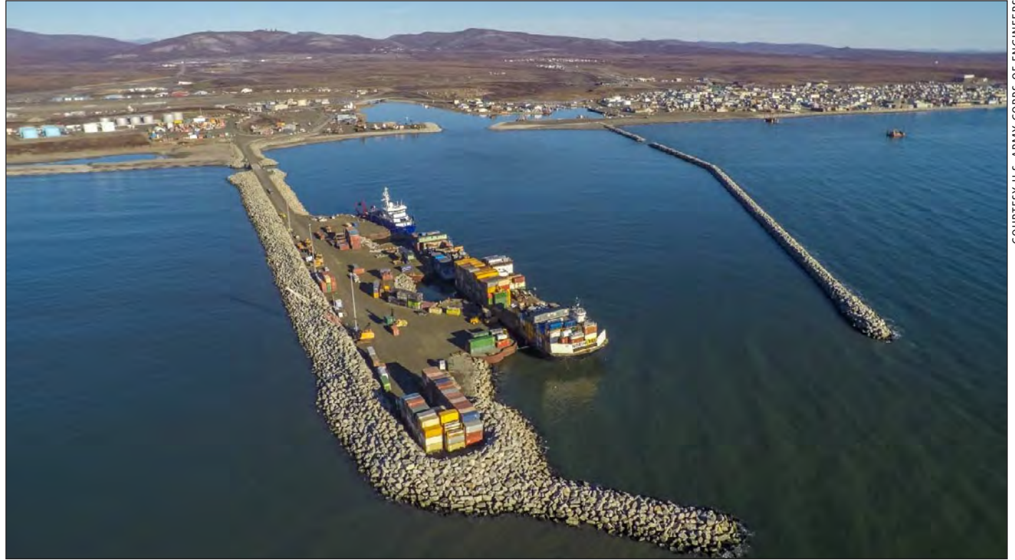
An aerial view of the Port of Nome. The proposed expansion involves adding a deep-water section beyond the current port entrance, deepening the existing outer basin and replacing the east breakwater.
