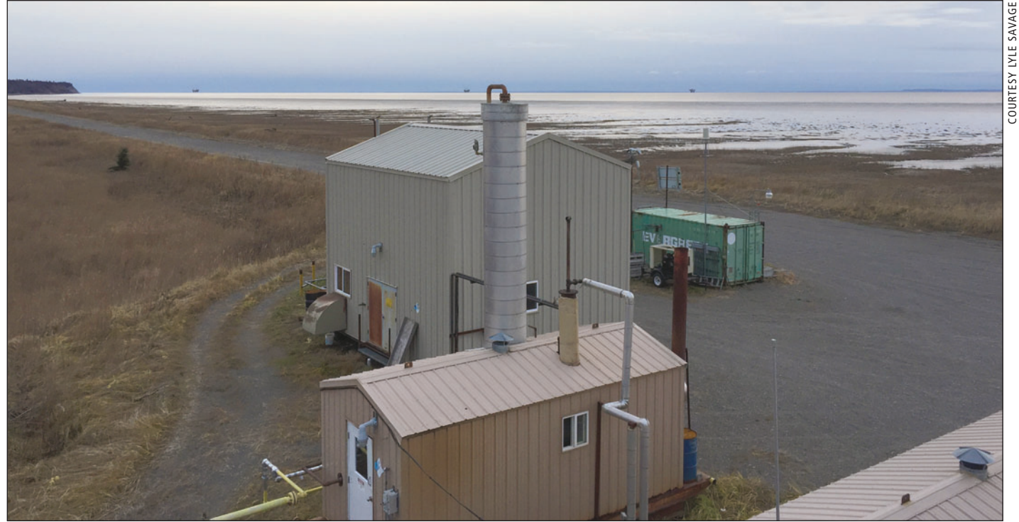
The compressor facility in Amaroq Resources' Nicolai Creek gas field.
