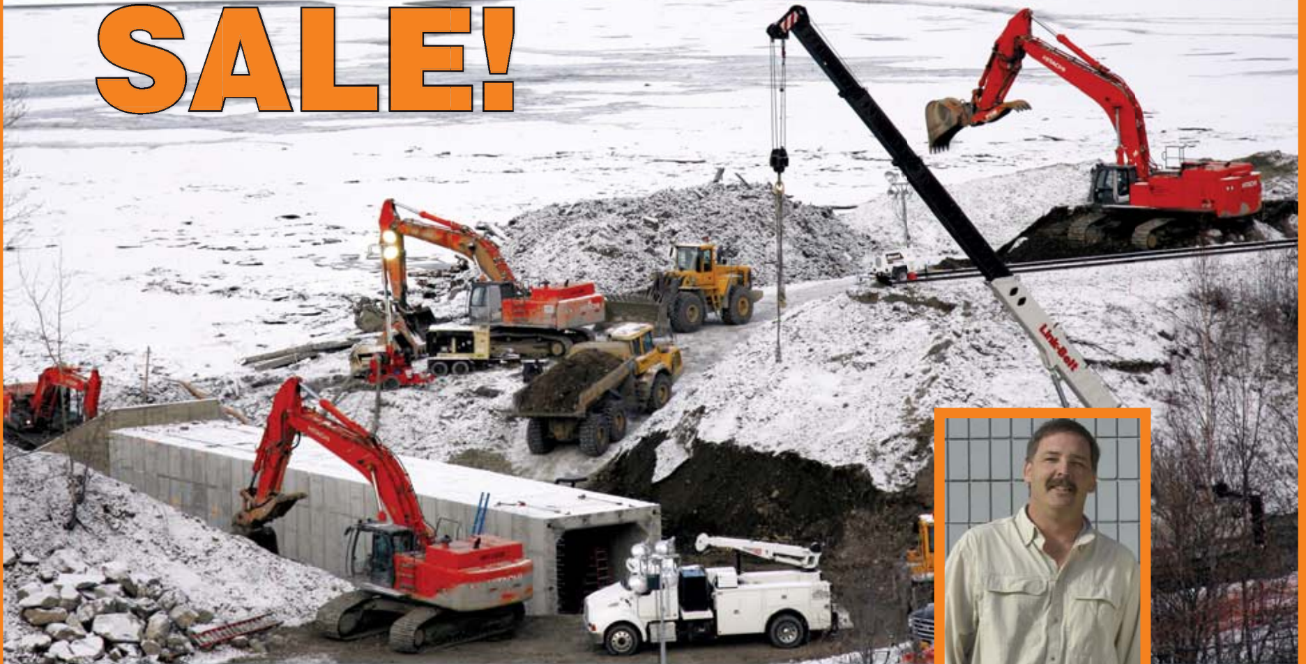
Above photo: Volvo, Hitachi, and Linkbelt equipment at the Hamilton Construction job site, Chester Creek, Anchorage
