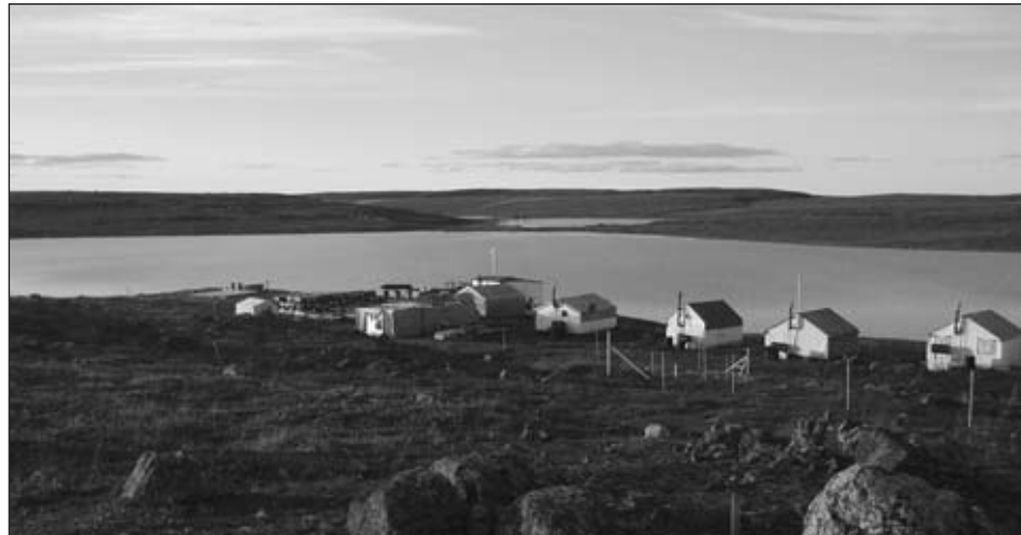
Sabina Silver drilled 43 holes covering 5,325 meters on its Hackett River property in Nunavut in 2008 from this exploration camp.
