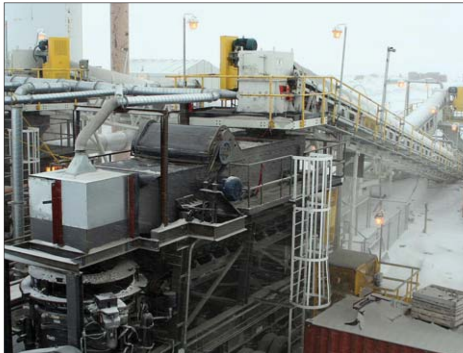
Mechanical issues at the Rock Creek Mine attributed to NovaGold's decision to suspend operations and place the gold mine near Nome, Alaska on care-and-maintenance.
