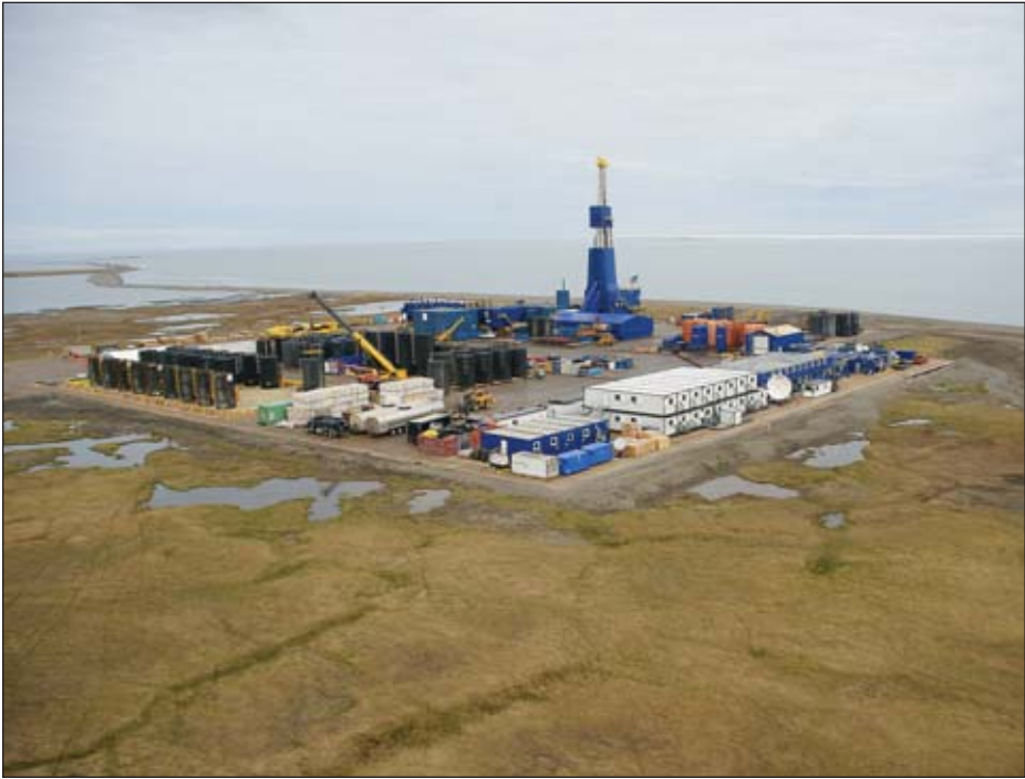
The Nabors 27E rig drilled the surface section of the second well at the Point Thomson central pad.
