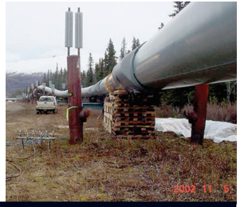
page 20 years ago: 7.9 quake shuts down 3 pipeline Nov. 3; up again Nov. 6
