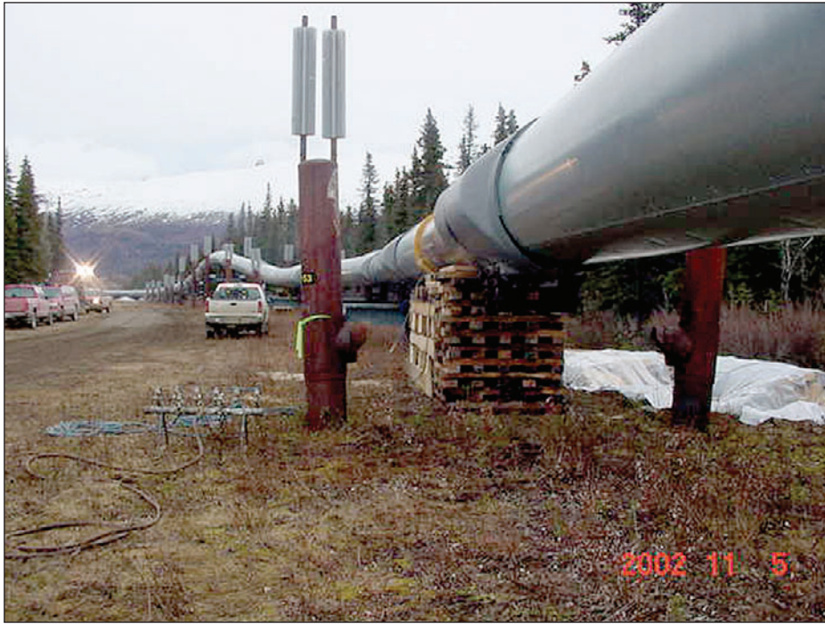
One of several “cribs” Alyeska Pipeline Service Co. installed under the trans-Alaska pipeline following the 7.9 earthquake which took place Nov. 3, 2002. Alyeska said the cribs are an industry-standard practice that helps support a structure like the pipeline — or a house that needs to be moved.
