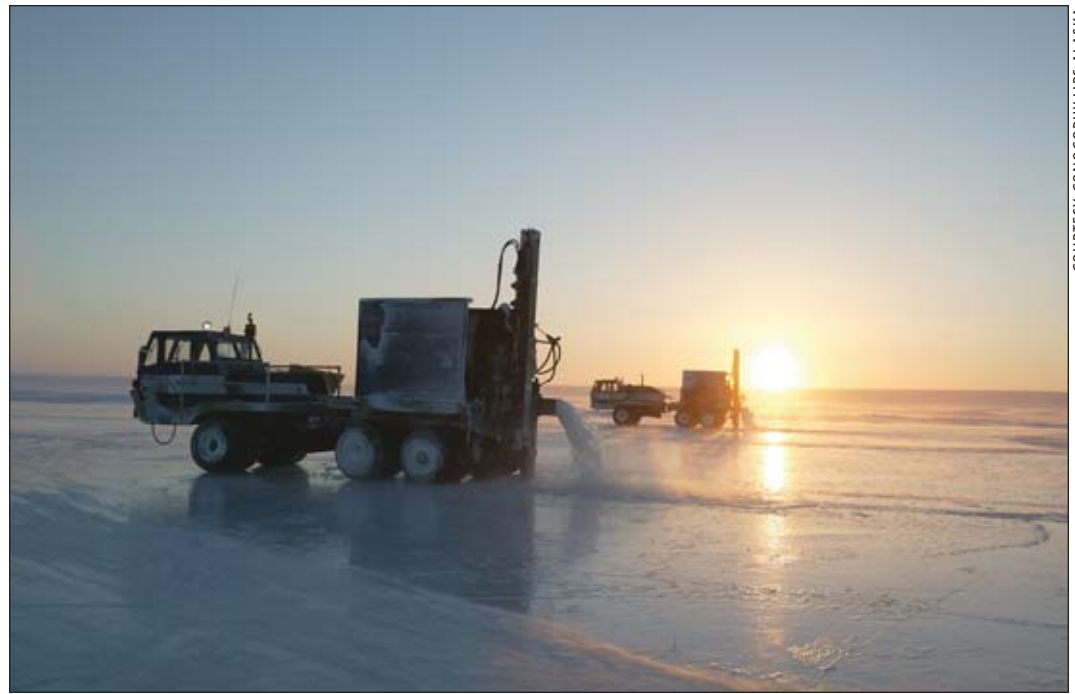
Building an ice air strip at Intrepid
