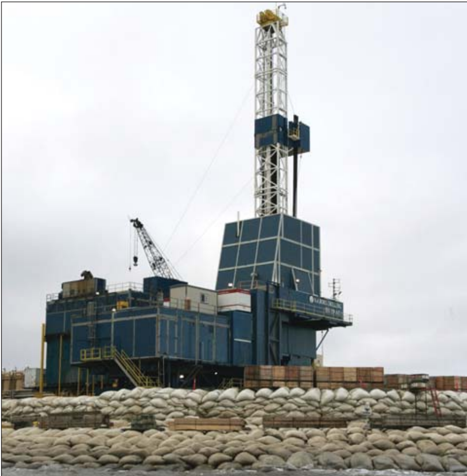
Nabors 19AC drilling rig
