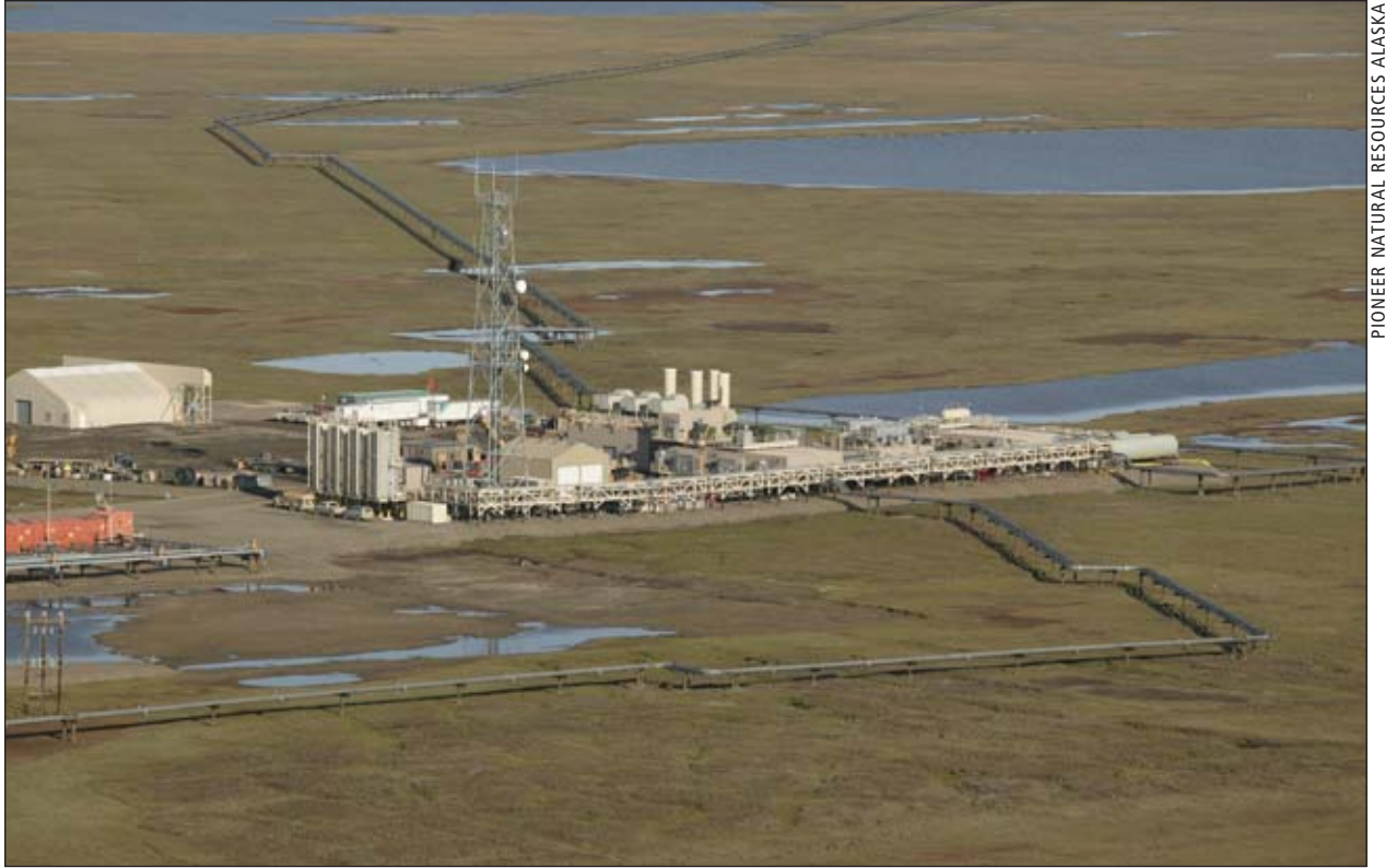
The Oooguruk tie-in pad at Kuparuk well pad 3H
