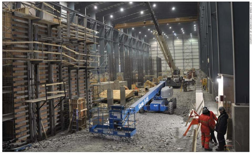
Construction crews prepare form work, front left, for concrete foundations in late March to support the semi-autogenous grinding (SAG) mill and the ball mill inside the Meadowbank ore processing plant. Projected mill recovery rates will range from 91 percent to 94 percent and mining/milling costs are expected to average C\$50 per metric ton for the Meadowbank gold project.
