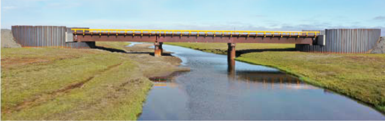
Miluveach River Bridge
