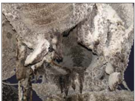
Looking up at the hole in the ruptured pipeline.
