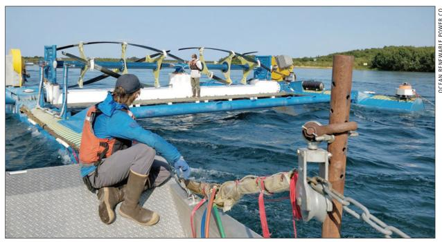
ORPC Engineers at work during retrieval and maintenance of the RivGen turbine generator at Igiugig.
