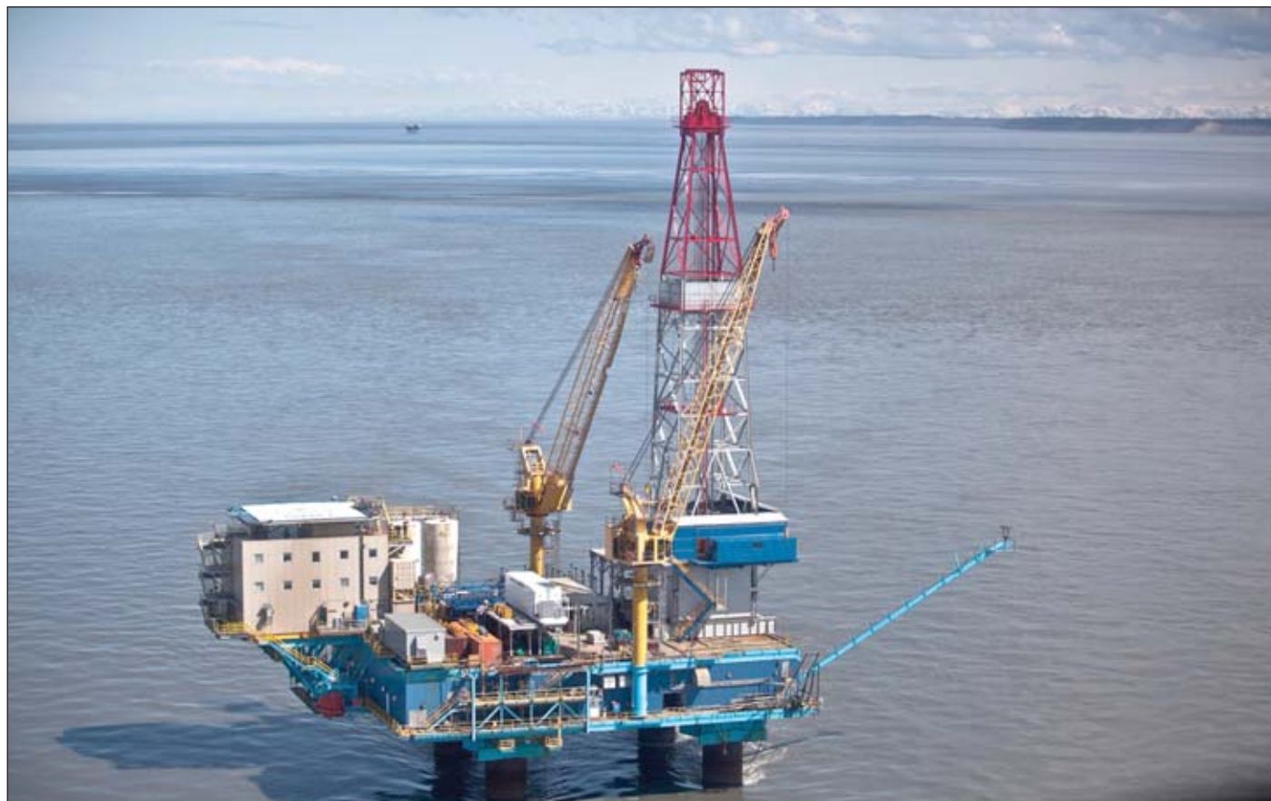
Cook Inlet Energy's Osprey Platform
