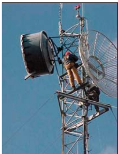
GCI technicians install and maintain the largest microwave (MW) network on the North Slope. GCI also owns and maintains substantial MW infrastructure throughout Alaska.
