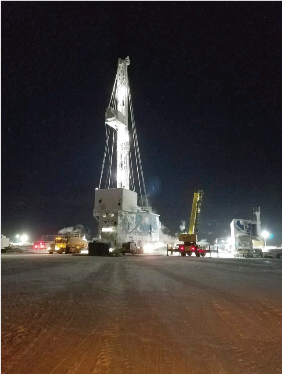
Rig 111 commissioning work in early January.
