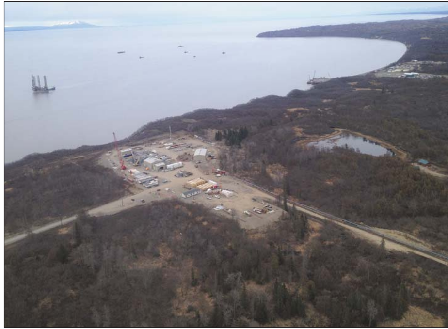
Furie Operating Alaska says that the onshore gas processing facilities, seen in the foreground, for its Kitchen Lights gas field are now 90 percent complete. The company's Spartan 151 jack-up drilling rig, seen in the background, is now in position for the operation of threading the field's gas gathering pipeline through an underground borehole to the onshore facilities.
