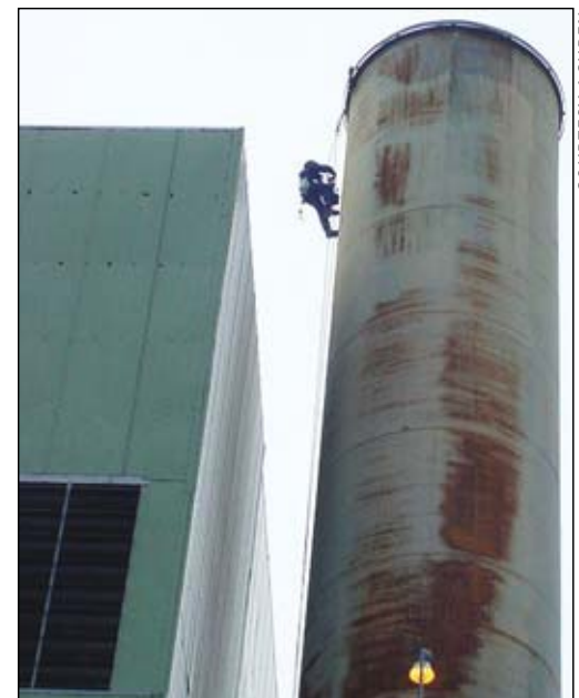
Acuren inspector using rope access technology to inspect a tower.
