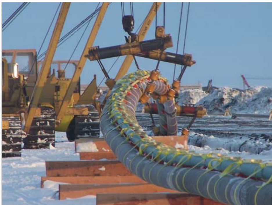
Lowering in Oooguruk offshore pipeline bundle.
