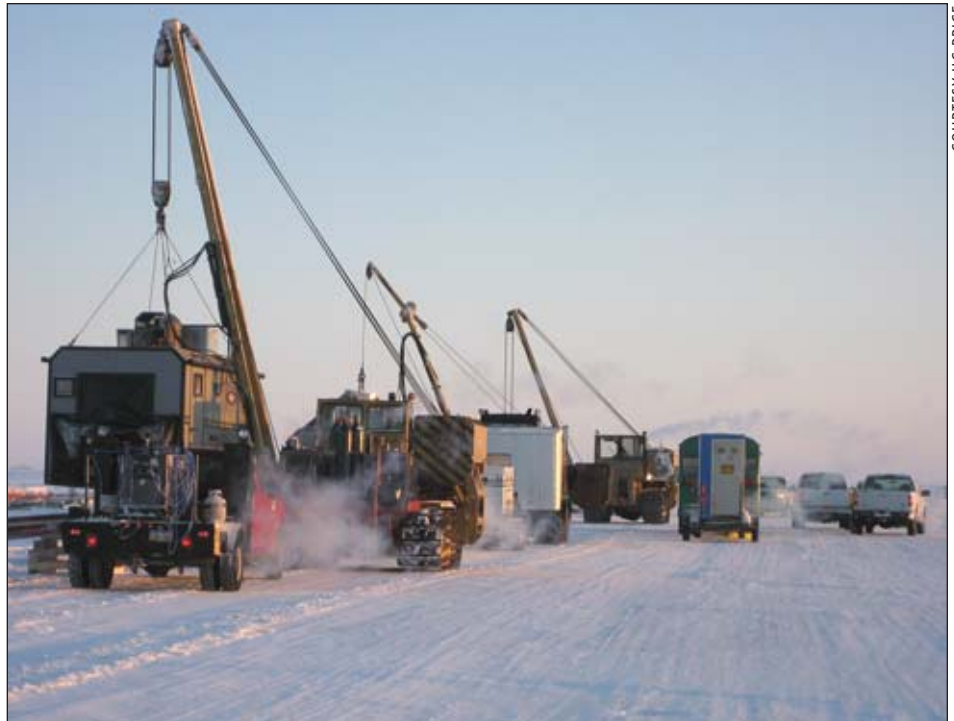
Setting vertical support members to elevation, North Slope
