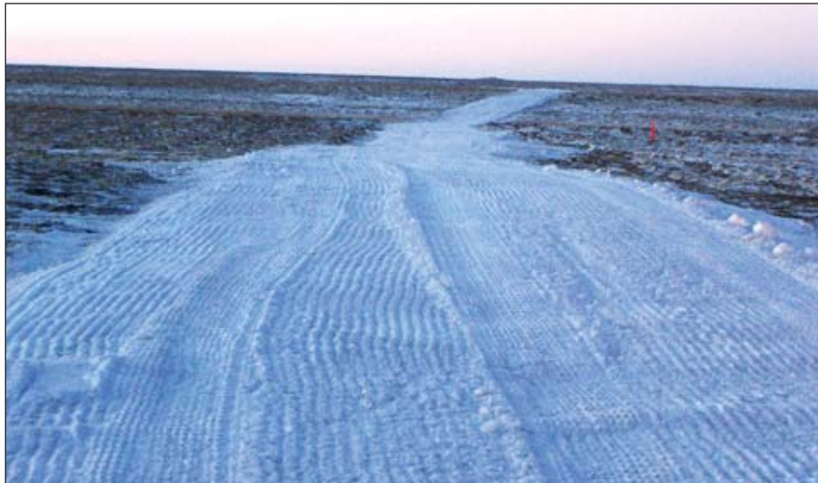
Pre-packing an ice-road route with snow and ice chips conserves snow, ready for road construction, as well as improving tundra protection.
