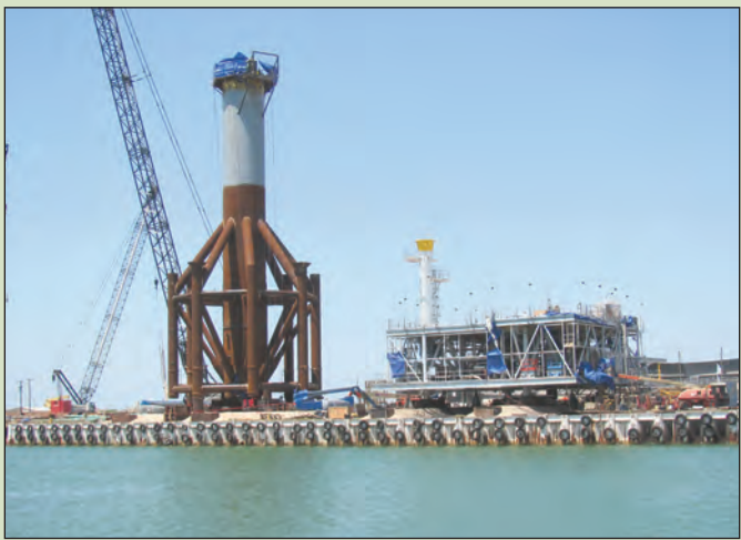
The monopod leg and platform for Furie Operating Alaska's Kitchen Lights unit A platform. The platform is soon to be shipped from Texas to Alaska's Cook Inlet.
