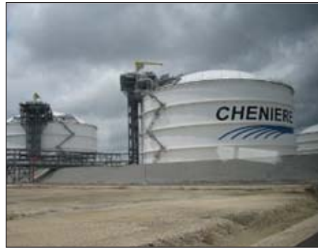
LNG storage tanks at Cheniere Energy's Sabine Pass, La., site.
