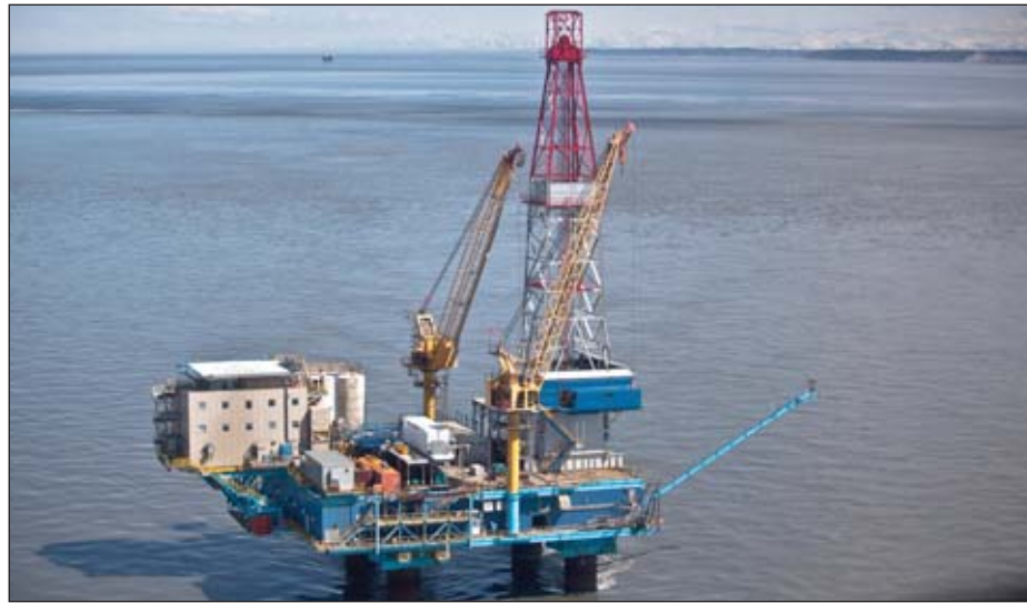
The new rig being assembled atop the Osprey platform.
