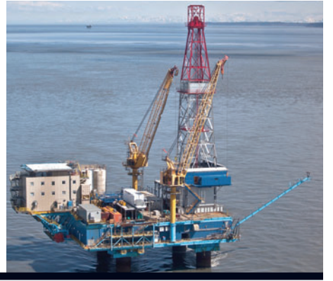
page 7 New rig going up on Cook Inlet Energy's Osprey platform in inlet
