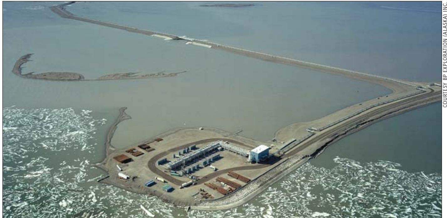
The Liberty wells will be drilled from this Endicott satellite drilling pad, expanded for the purpose. The pad is connected to the shore by a causeway.
