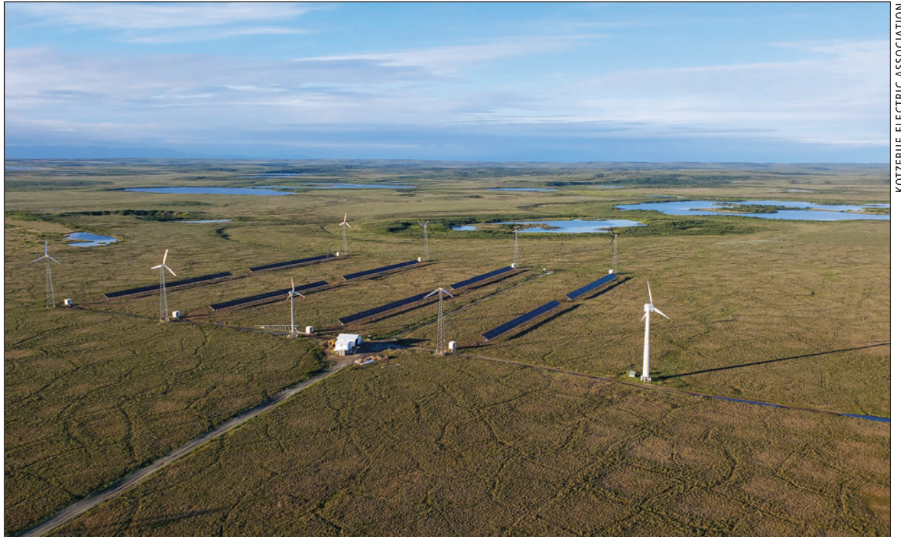
Kotzebue Electric Association's solar and wind farm. Advanced technology integrates wind and solar energy with diesel generation and battery storage to reduce diesel consumption.
