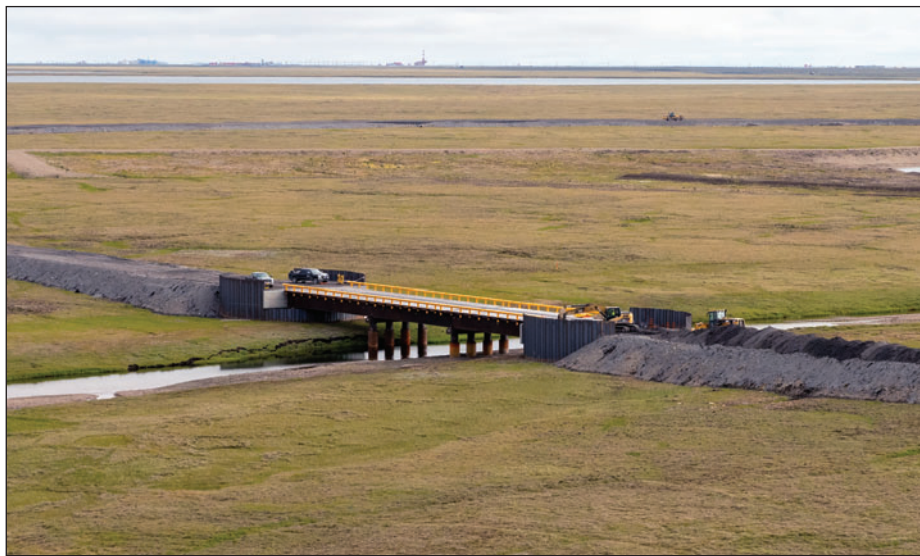
Oil Search's summer work program included bridge installation across the Miluveach River.
