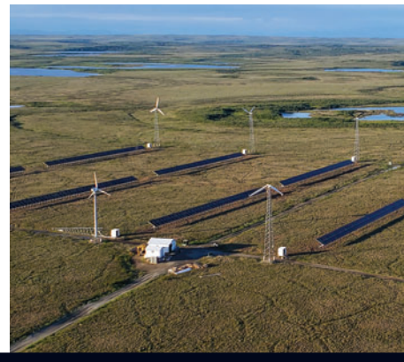
page 2 With 200 installed, rural Alaska leads way for microgrid systems
