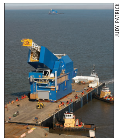
In August, being delivered to the North Slope at West Dock, is Parker Drilling's Rig 273 drill module. The two rigs' utility modules and the Rig 272 drill module are on the barge in the background.
