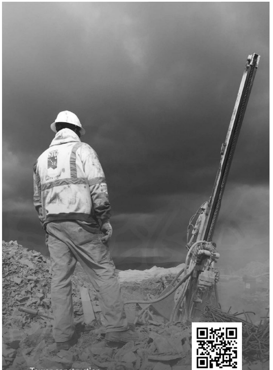
Tower construction along the Yukon River.
