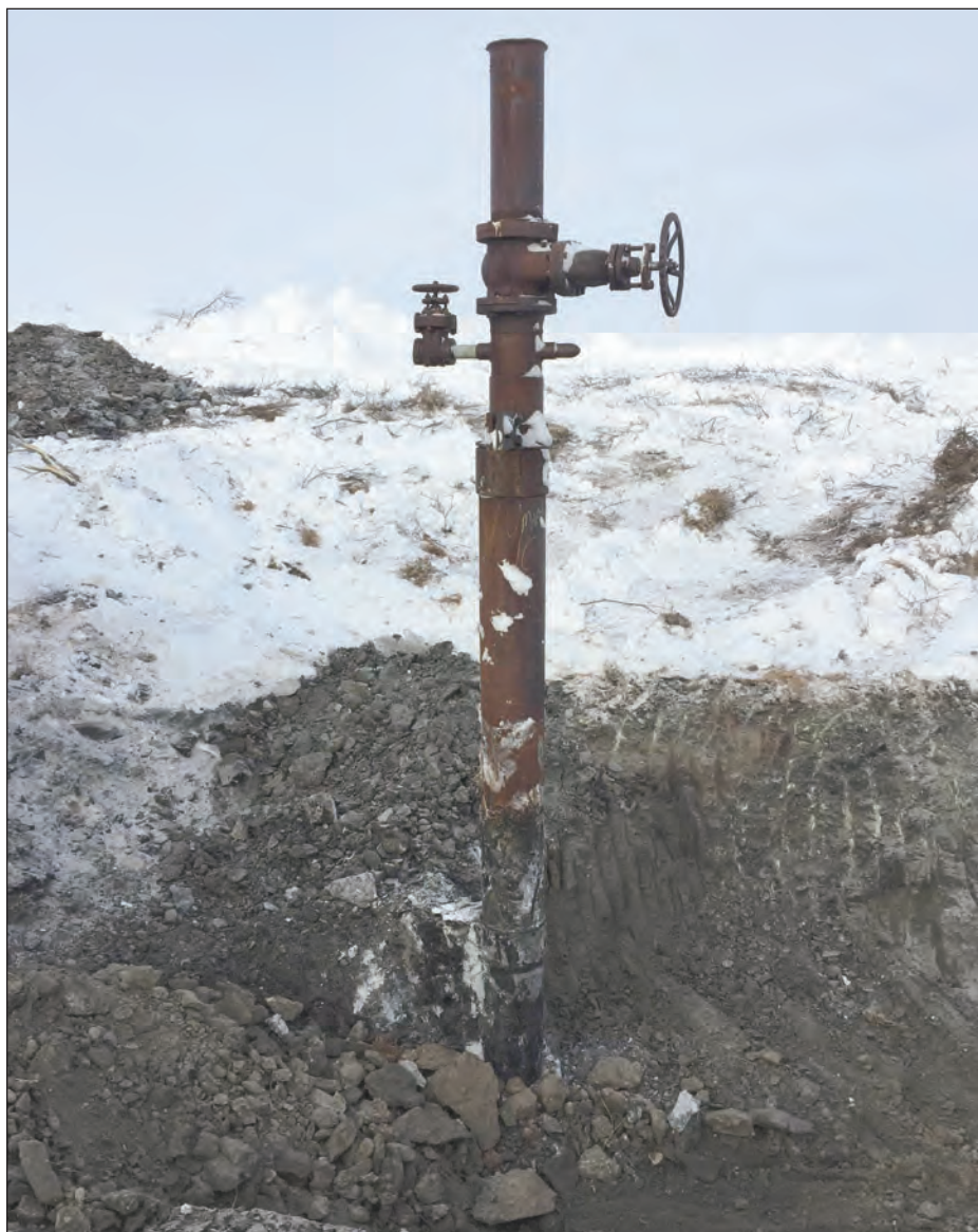
Umiat No. 10 was excavated for removal of the wellhead.
