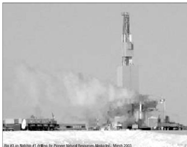
Rig #3 on Natchiq #1 drilling for Pioneer Natural Resources Alaska Inc., March 2003
