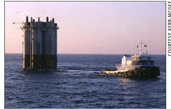
A recent photo of Red Hawk, the world's first cell spar, which Kerr-McGee is using to develop the Red Hawk field in 5,300 feet of water. Red Hawk was upended this month. The topsides are in route and could be set by month-end.
