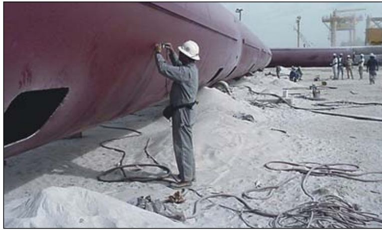
Exxon Diana Hoover platform buoyancy can coating being inspected in vendors yard by NACE coating inspector
