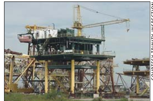
An offshore platform dry-docked for refurbishment — Trinity Inspection Services monitors all phases of platform maintenance, coating and welding inspections and corrosion surveys.
