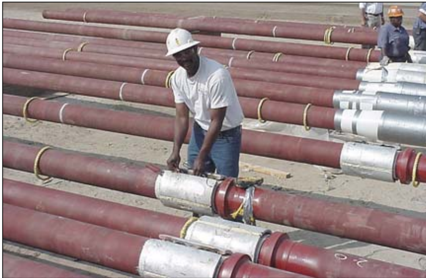
NACE coating inspector performing continuity test on a 16-inch pipe anode
