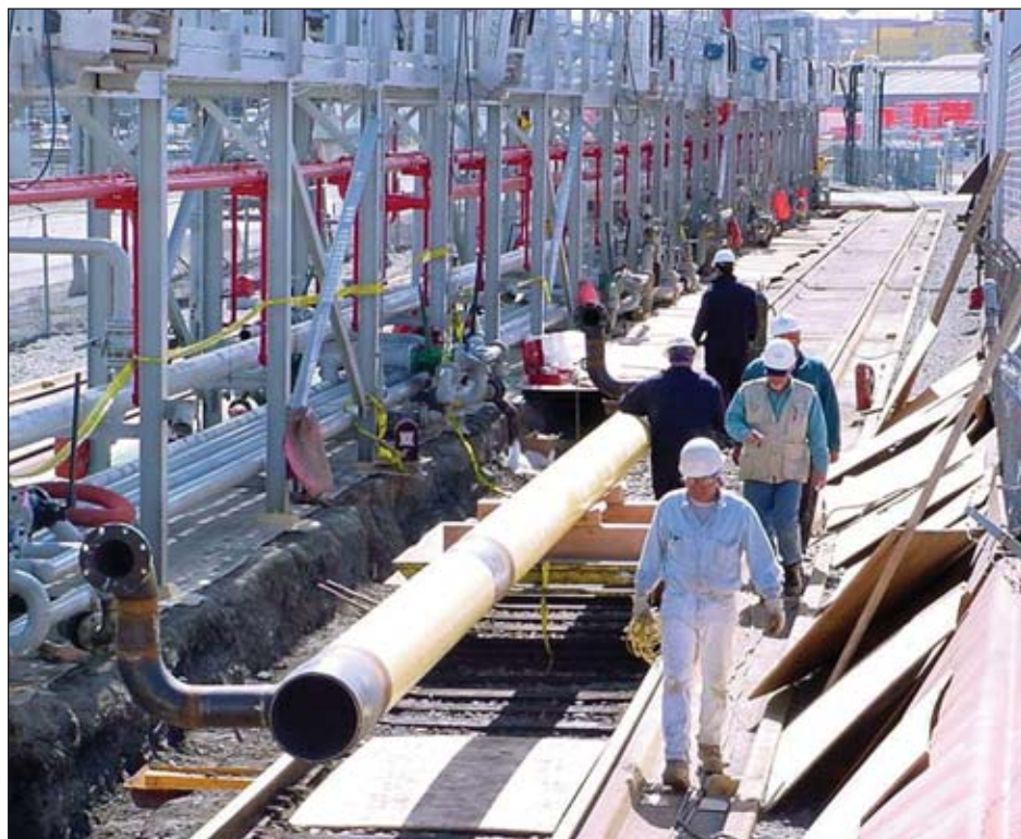
Udelhoven's railcar rack expansion at Port of Anchorage
