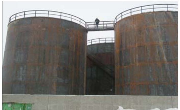
Mark Helmericks, Colville president and CEO, on the catwalk inspecting the tanks.
