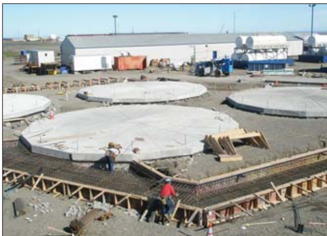
Foundation work under way.
