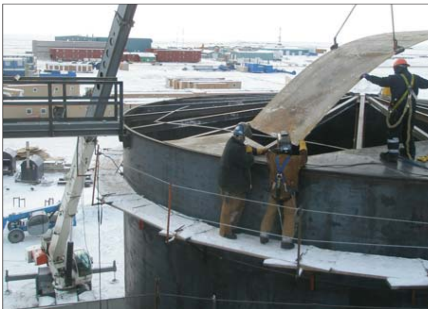
Installing roof sheets on one of the tanks.
