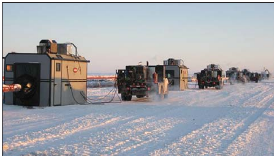
PGI-designed welding shelters that exhaust smoke and improve welders' breathing environment and productivity.
