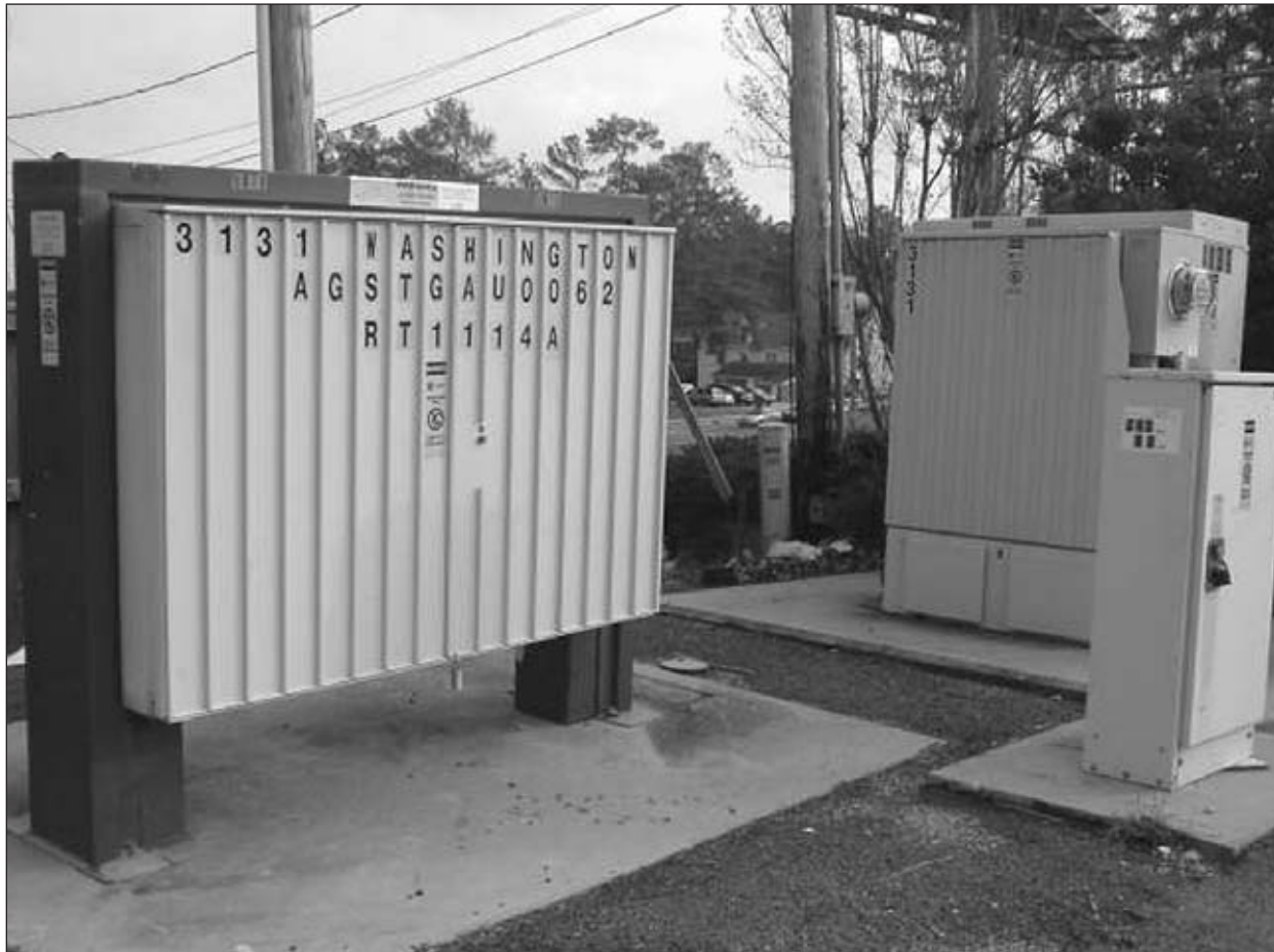
Transformers, like these, used in telecommunications, utilities, transportation systems and other public institutions are increasingly tempting targets for copper theft.
