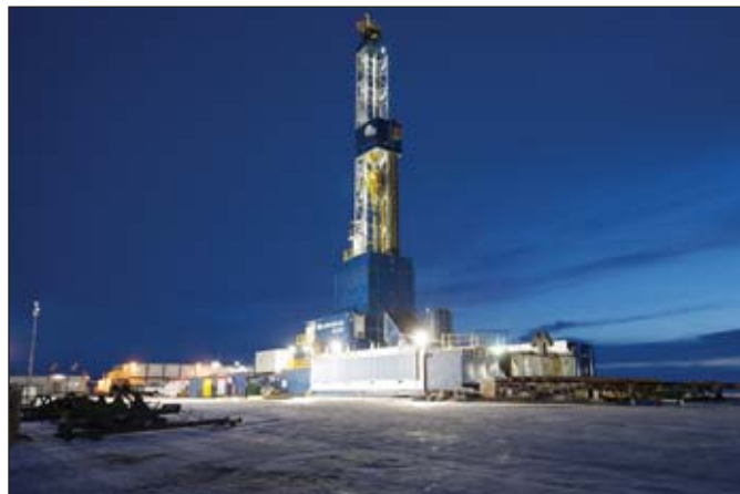
Another first in a year of major milestones is Anadarko Petroleum's natural gas exploration project in the Gubik field, south of Prudhoe Bay.
