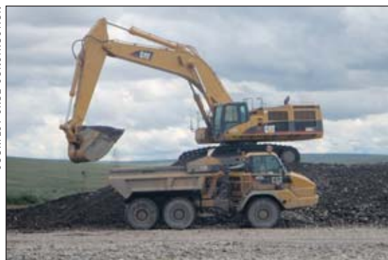
CAT 385 Stockpiling Gravel at Happy Valley
