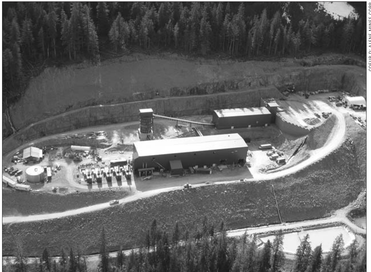
Coeur Alaska has spent more than $230 million building the proposed Kensington gold mine near Juneau, Alaska. The company is waiting on the U.S. Supreme Court to rule on its tailings disposal permit.
