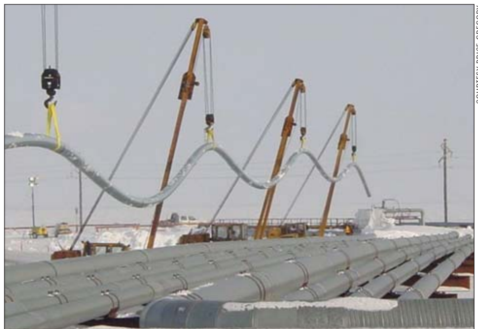
Coordinated lift over live pipelines for raise-up of new water injection pipeline replacement at Kuparuk.
