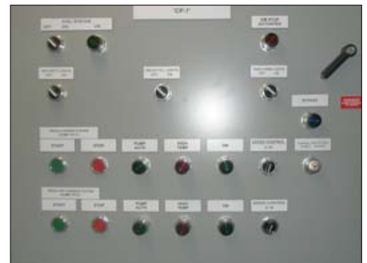
Tank farm's control panel.
