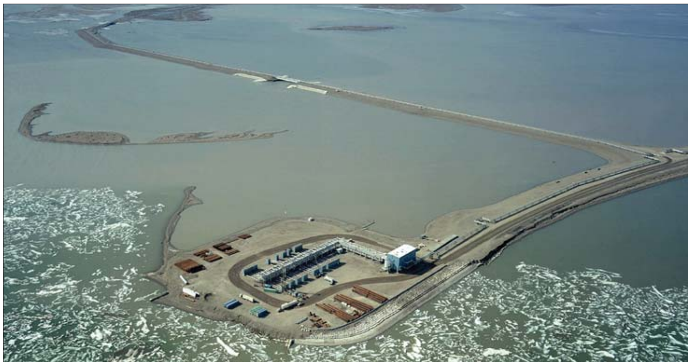
The Liberty wells will be drilled from this Endicott satellite drilling pad, expanded for the purpose. The pad is connected to the shore by a causeway.
