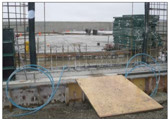
In this photo you can see how high the concrete revetment walls are.
