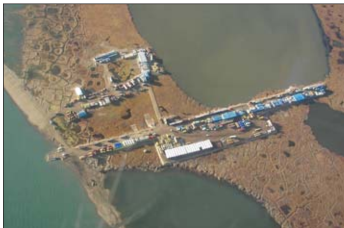
Three days after completion, the client, FEX, had a functional pad for staging materials and equipment.
