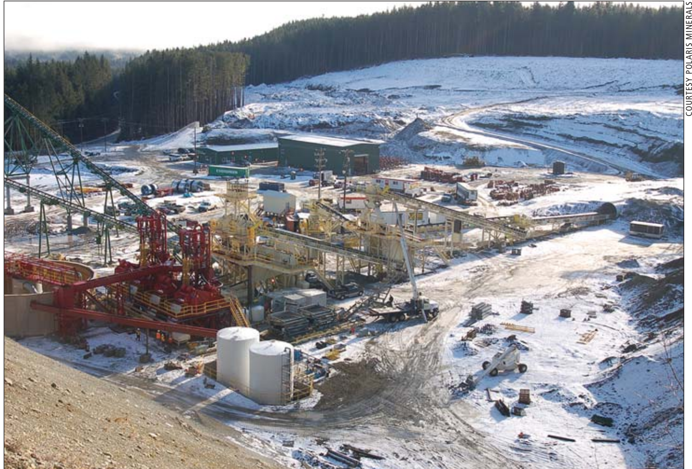
The Orca sand and gravel deposit can be seen in the background of this view of the quarry.
