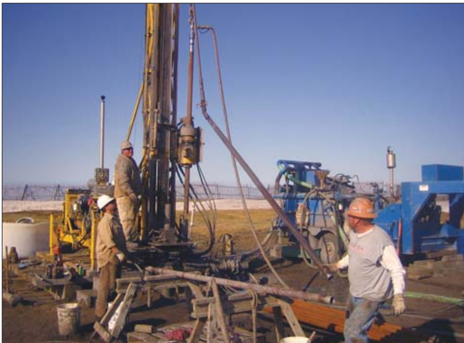
Removing the core barrel inner tube from the Wainwright coalbed methane test well
