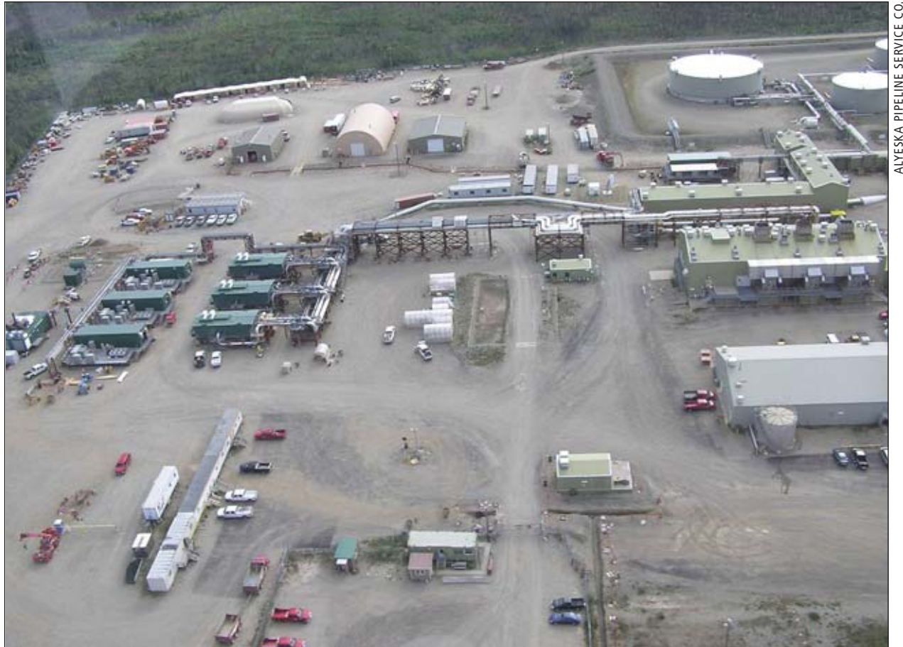
An aerial view of pump station 9. The train of three new electric pumps and associated variable frequency drives can be seen in the middle left part of the picture. The site layout includes space for additional pumps should Alyeska need to up the maximum pipeline capacity.
