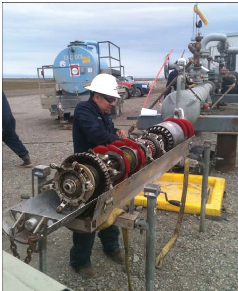
A technician prepares a smart pig for launch down the Badami oil pipeline, to check the pipeline prior to restart.
