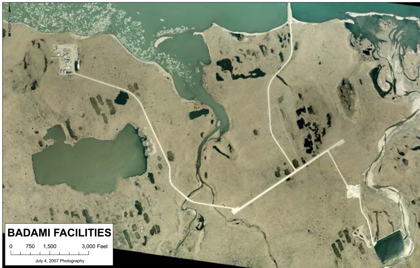
The Badami pad and central processing facilities.
