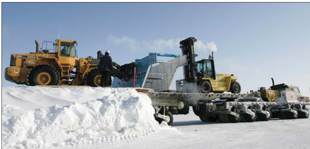
Unloading part of a drilling rig and a forklift onto a ramp made of ice and snow at a remote location
