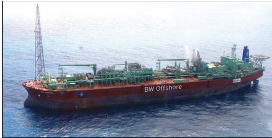
BW's Yuum Kak Nabb FPSO undergoing installation in the Bay of Campeche on Mexico's side of the Gulf of Mexico. A similar FPSO will be installed at Cascade-Chinook on the U.S. side of the Gulf.
