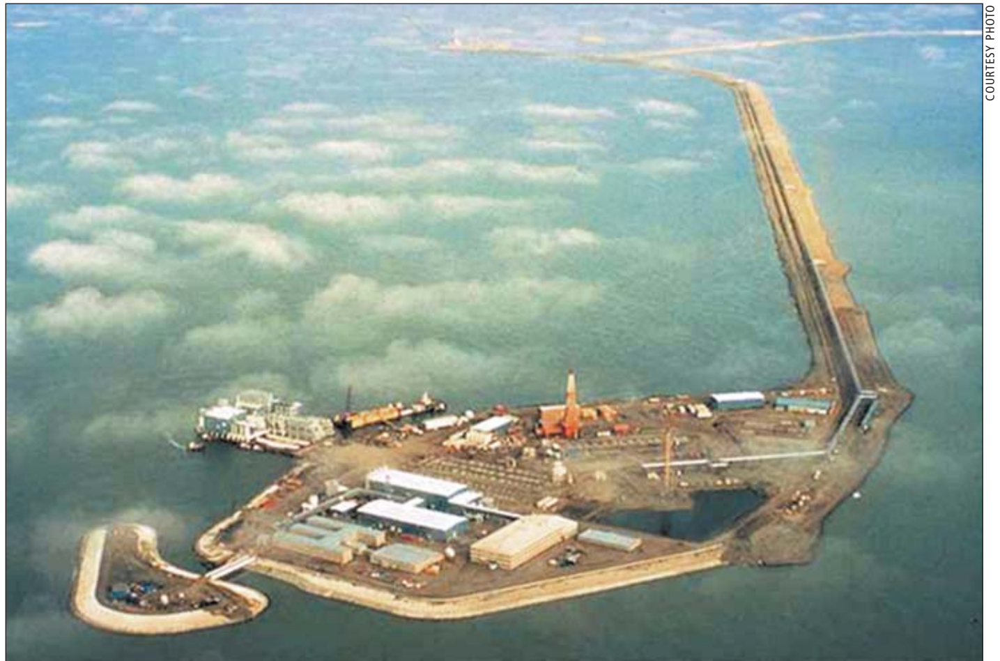
Alaska holds the honor of producing the first oil from Arctic waters: BP’s Endicott oil field in the Beaufort Sea. Northeast of Prudhoe Bay, Endicott is connected to the mainland by a 1.5-mile gravel causeway.
