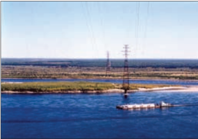
Power lines in the Sakha Republic (Yakutia), Russia
