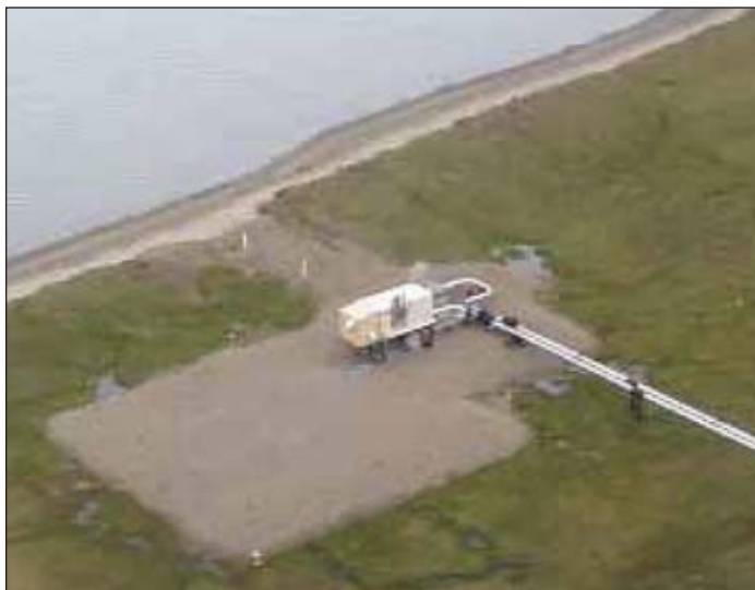
Aerial view of the Northstar shore crossing landfall at Point Storkersen, the point where the pipelines transition between buried sub-sea and supported above-ground. The visible module houses an RTU valve.
