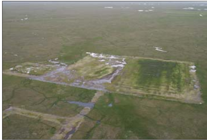
North Slope operators agreed to clean up and rehabilitate reserve pits where they once deposited drilling waste. With the help of industry and state biologists, this reserve pit is well on its way to being reclaimed by the tundra.
