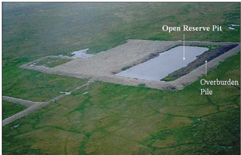
Reserve pits on production pads like this one built in 1978 were an integral part of drilling waste management practices on the North Slope until the 1980s.
