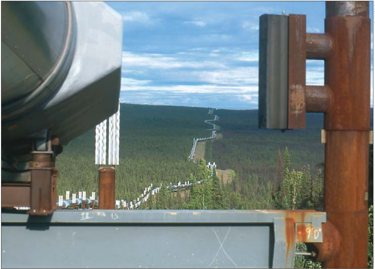
The 800-mile trans-Alaska pipeline system starts at Prudhoe Bay and terminates at the Port of Valdez.
