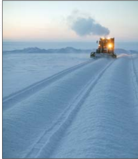
Making ice chips for building ice roads
