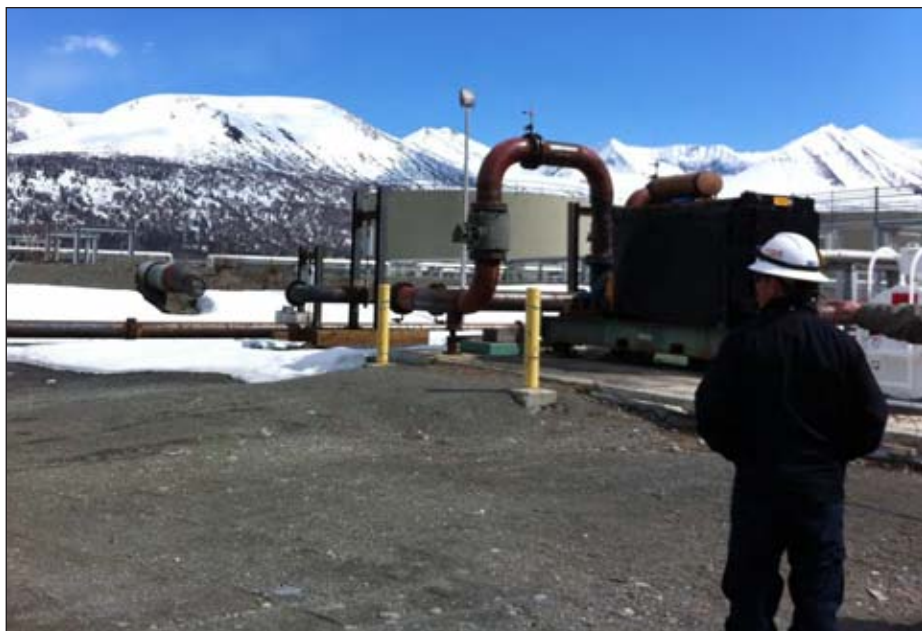
A staff member from the State Pipeline Coordinator's Office views pump station 12 modifications designed to facilitate a cold pipeline startup in the winter.
