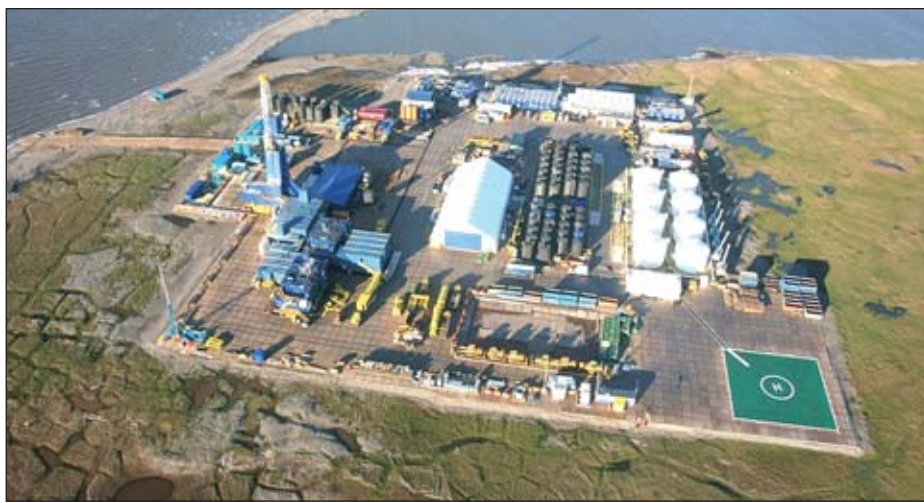
Point Thomson is a remote natural gas and condensate field approximately 60 miles east of Prudhoe Bay.
