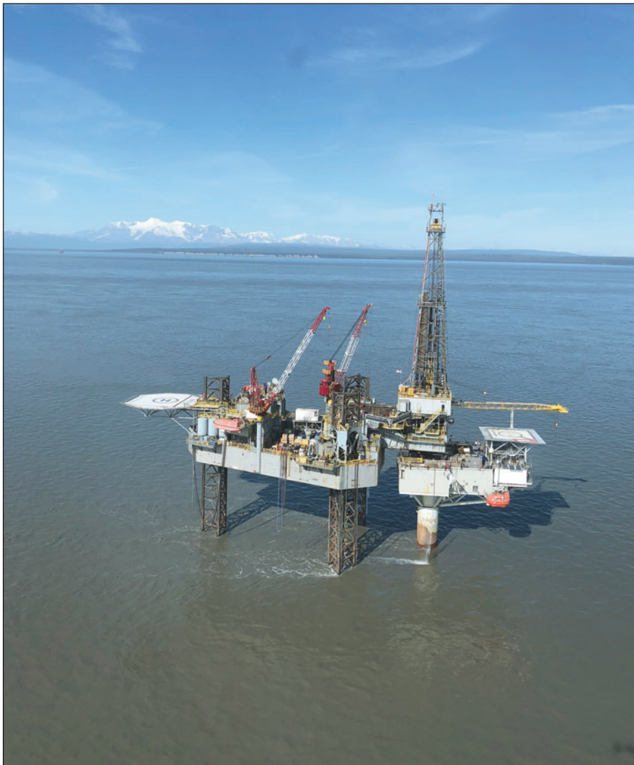
The Spartan 151 jack-up rig cantilevered over the Julius R platform for development drilling in the Kitchen Lights gas field in Cook Inlet.
