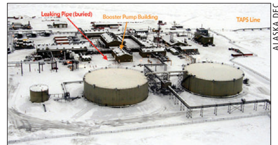
Aerial View of Pump Station 1 showing location of booster pump building and leaking pipe.
