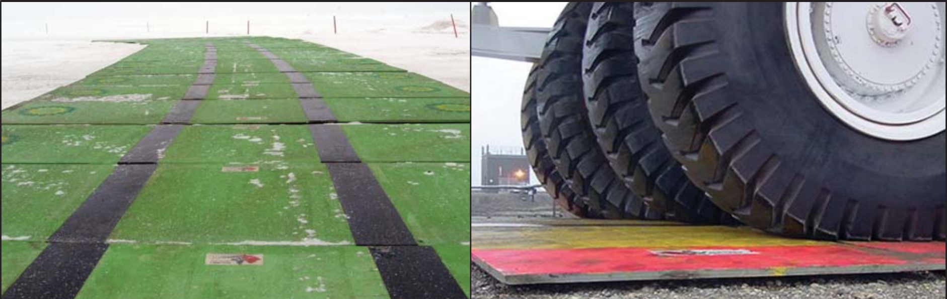
Tuvvaq Mat — on deteriorating ice road
