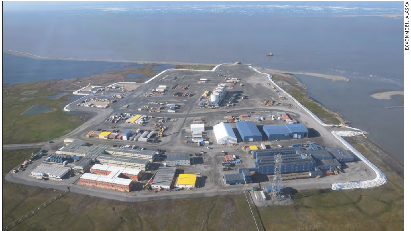
The Point Thomson central pad in August 2014. The permanent operations camp on the pad has been completed, as has the installation of diesel fuel tanks. The major facility modules are scheduled to arrive by barge in the summer of 2015, with smaller modules to be transported by truck from Anchorage in the winter of 2014-15, using a winter ice road to reach the field site.
