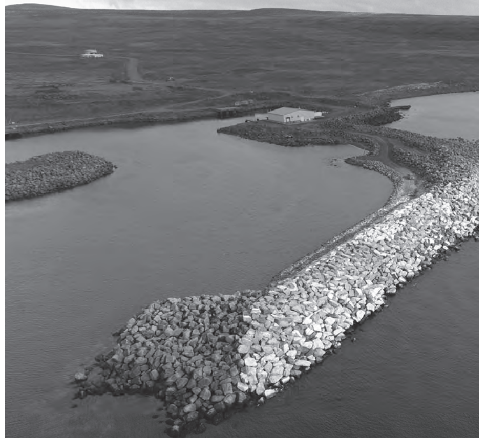
Saint George, Alaska storm repair post-construction aerial inspection.
