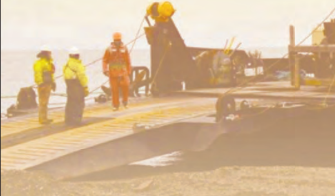
Brice Marine - Wainwright Seawall Construction Wainwright, Alaska
