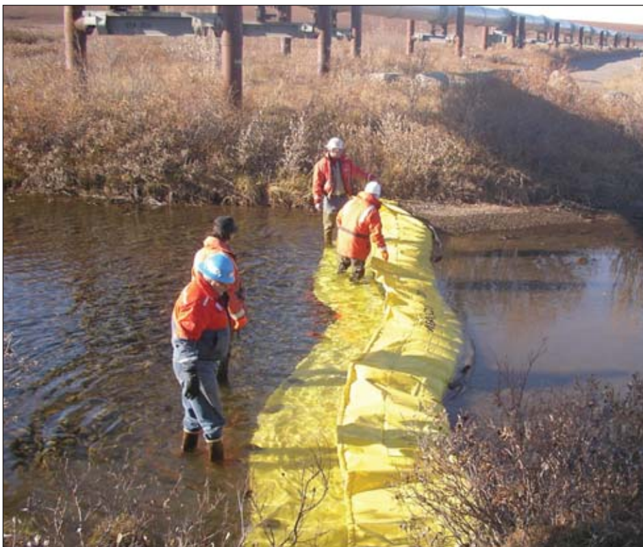
Two workers can deploy this 100-foot, 68-pound water dam in five to 10 minutes to do the work of a sandbag dam that would take at least two hours to erect with at least three times the manpower. Alyeska Pipeline Service Co. purchased the technology from a French manufacturer called Megasecur.
