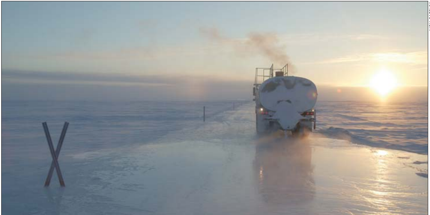
Building an ice road by applying water from a water truck
