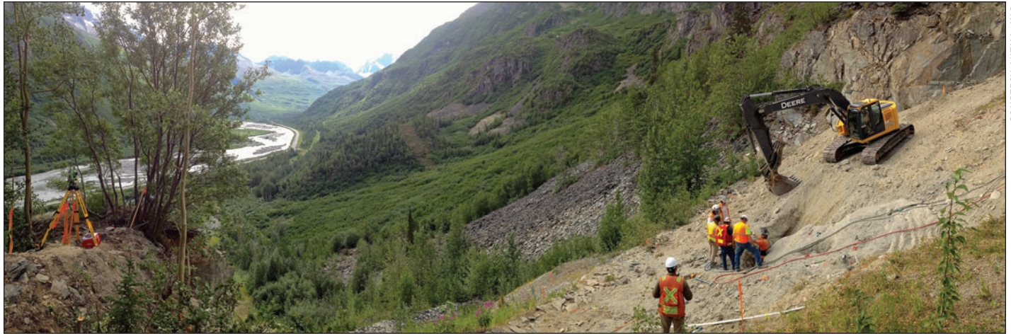
An Ahtna Construction & Primary Products Company crew performs mainline integrity investigations on the Trans-Alaska Pipeline at Milepost 756.74.
