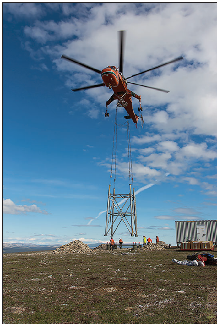
A heavy-lift helicopter lowers a section of a mountaintop GCI TERRA tower into place.
