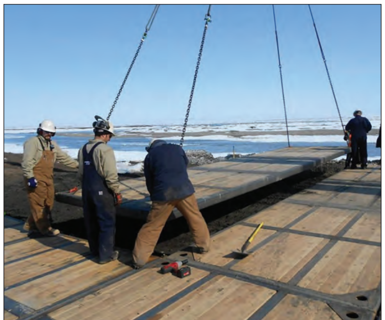
Rig mats being installed on the North Slope.
