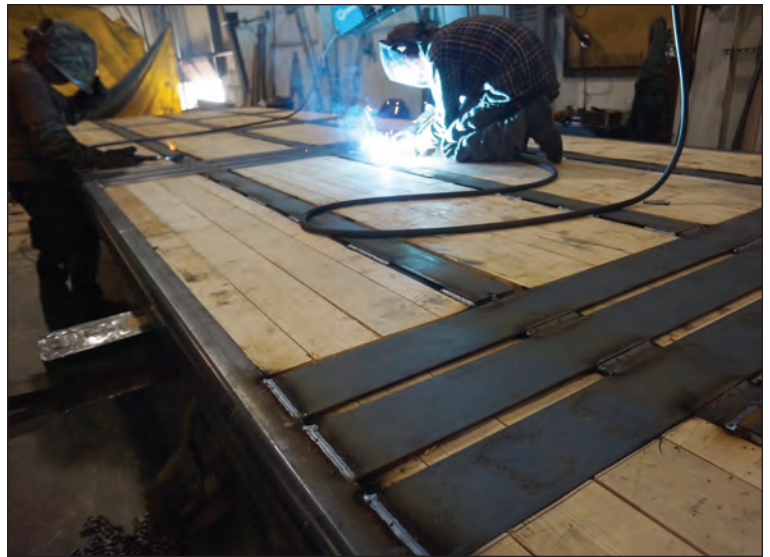
Four rail rig mats being reinforced.
