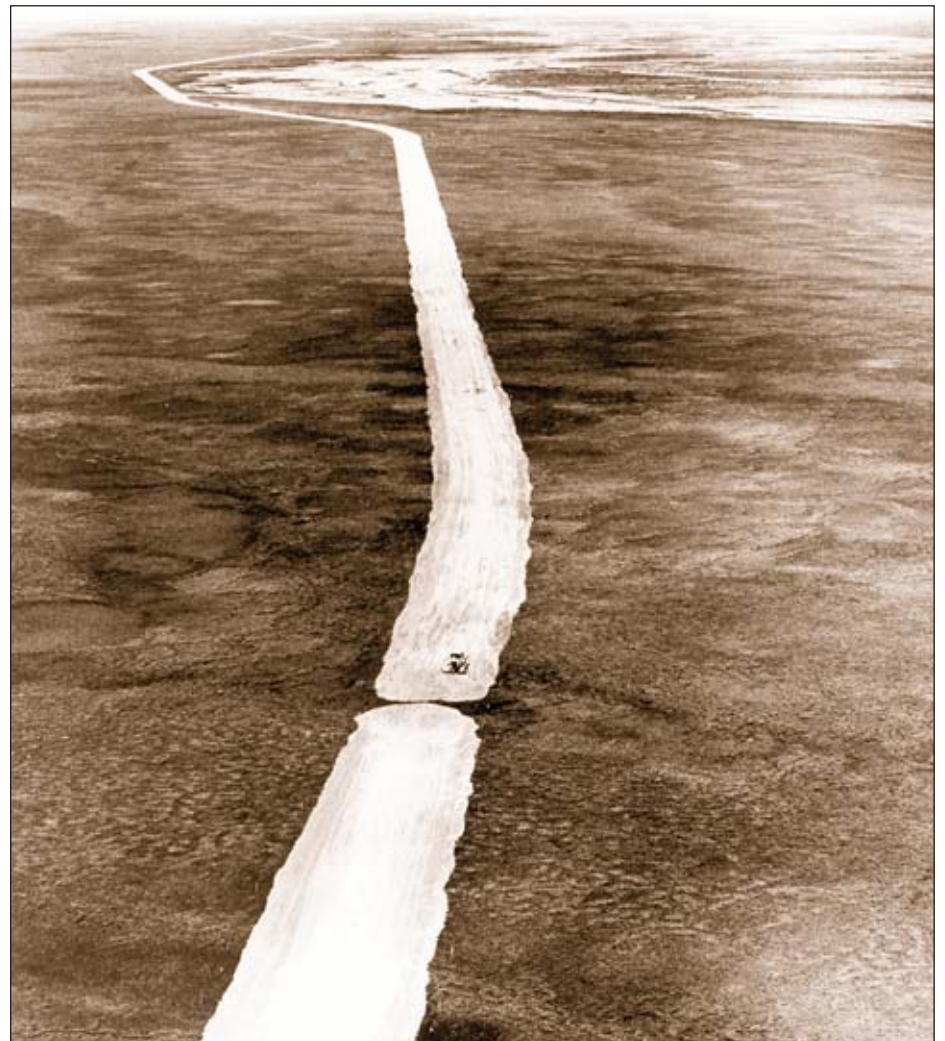
Haul road linkup: One of the first linkups of the 360-mile Prudhoe Bay to Yukon River highways occurred when construction crews working from the north and south met at this site on the tundra between Prudhoe Bay and Franklin Bluffs construction camp. A total of 32 million cubic yards of gravel were required to build the road.
