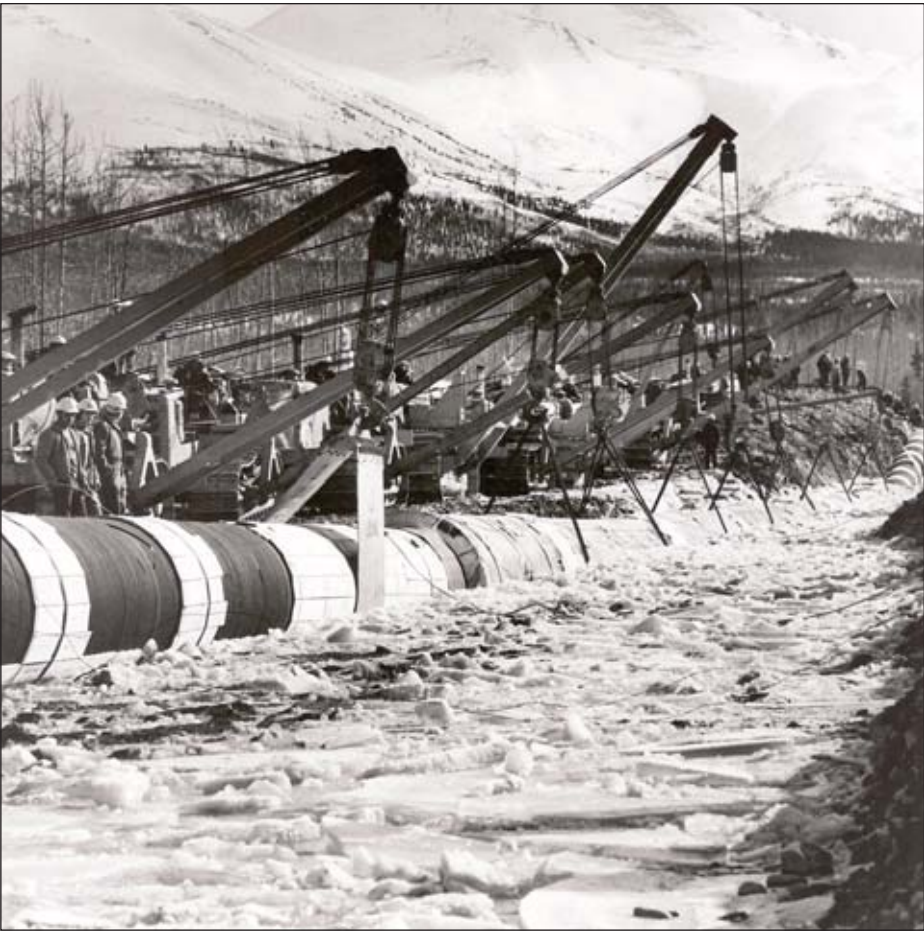
First installation was at Tonsina River in the spring of 1975. The pipe was weighted with concrete anchors for burial below the river bed.
