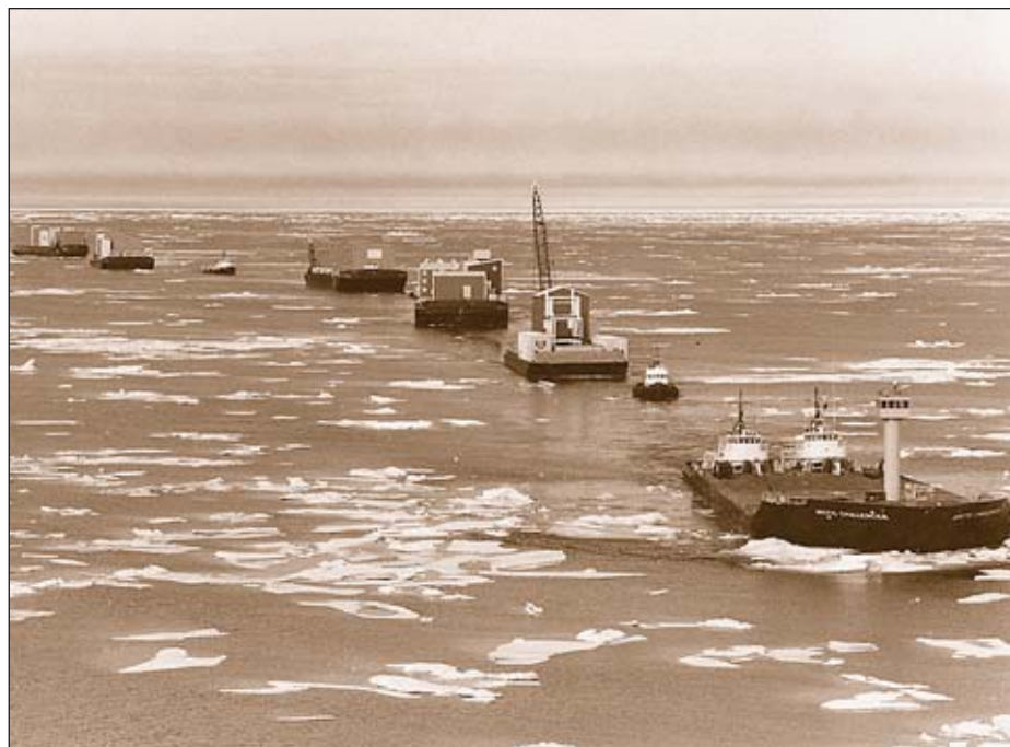
After a sea-journey of 3,000 miles from the U.S. West Coast, BP's 1975 sealift arrives at Prudhoe Bay with critically needed modules and equipment.
