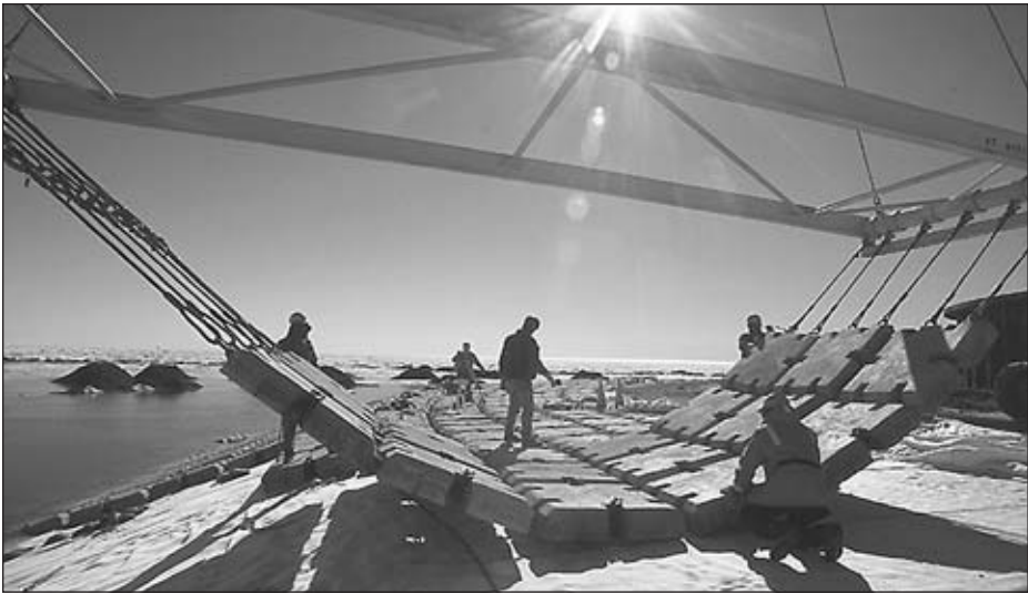
Alaska interstate construction crew laying mats for slope protection at Northstar Island June 29, 2000. Underwater divers complete the process of linking the mats together.
