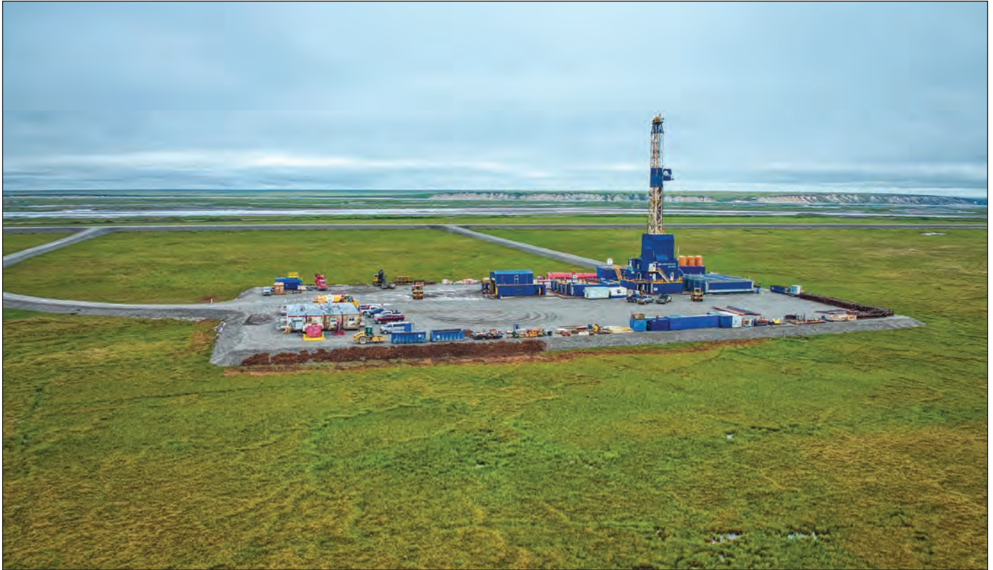
Nabors 105AC rig drilling Alkaid 2 well.
