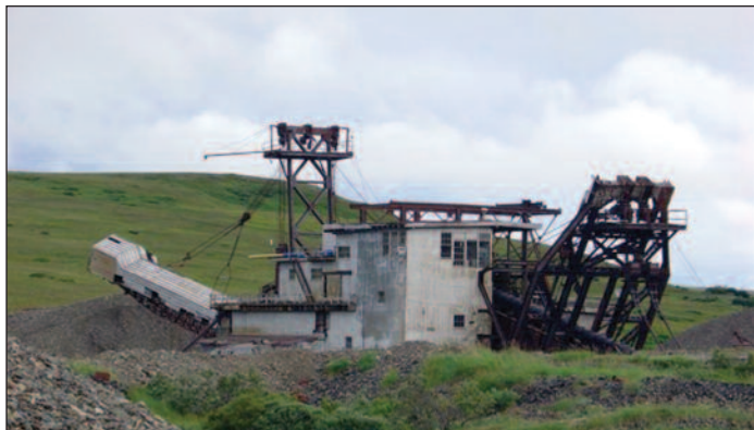
This dredge, put into operation by Goodnews Mining Co. in 1937, recovered the majority of the 650,000 of platinum extracted from the Salmon River area of Southwest Alaska. Courtesy of Calista Corp.
