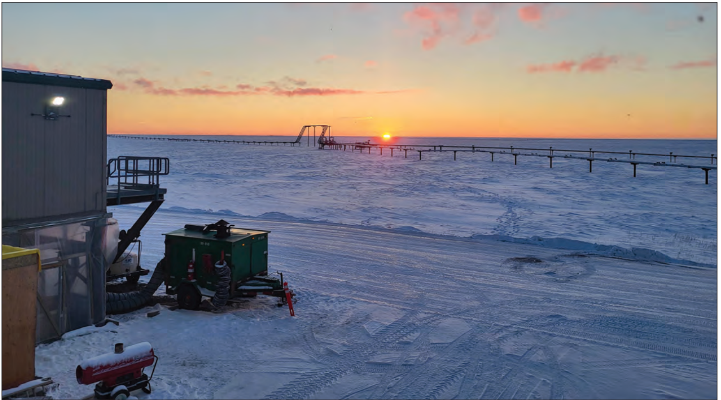
The sun rises on the Southern Miluveach unit connection to the Alpine pipeline.
